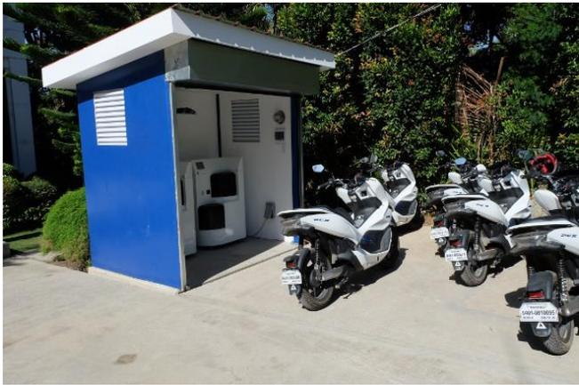
Figure 3: E-scooter battery exchange station (Topgear 2019)
